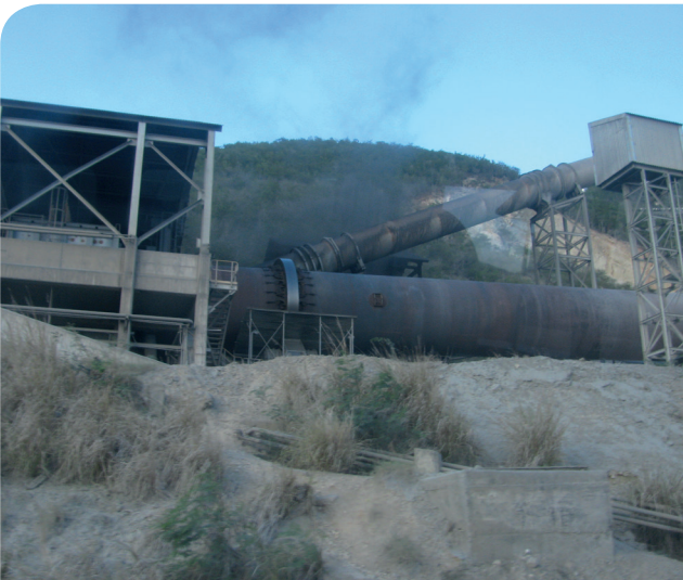
Coal dust emission from fine coal bin.
