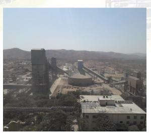
**PENTA** provided complete engineering of a slag grinding unit for a major steel processing company in India. The company plans to utilize its significant slag reserves in the manufacturing of slag cement under government sustainable development folio. PENTA's battery limits for the project started from the receiving of raw materials to packing and dispatching the finished product in small bags and bulk bags. PENTA prepared а technical/economic feasibility study, and completed basic
