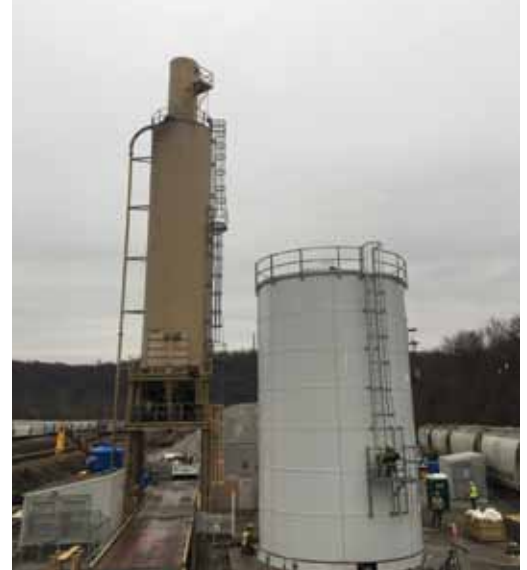
Figure 1: new bolted silo at mid-height
