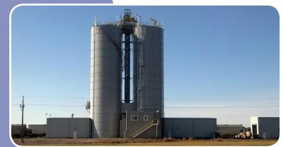
completed and fully operational within 3.5 months, prior to availability of site utilities. Power and compressed air supply needs were met with portable modular systems configured by PENTA. The main terminal consisting of rail car unloading, bulk storage, office/control building and truck loading system was completed within 10 months using extensive prefabrication and modular designs. The secondary system also handles alternate materials and can be used as a back-up.
